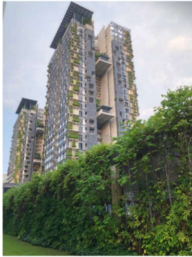
Two of the residential tower blocks at Kent Vale
