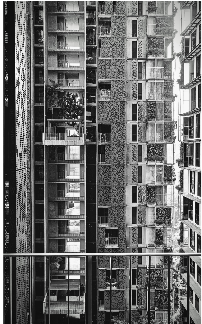
Figure 1: Looking towards Block H from Block G within Kent Vale. I really enjoyed the architecture here, the use of plants all over the building, the inside-outside gaps on every floor, and the wonderful rooftop terrace.
